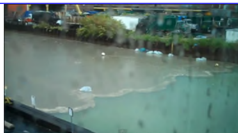
This is what Combined Sewage Overflow (CSO) can look like.
